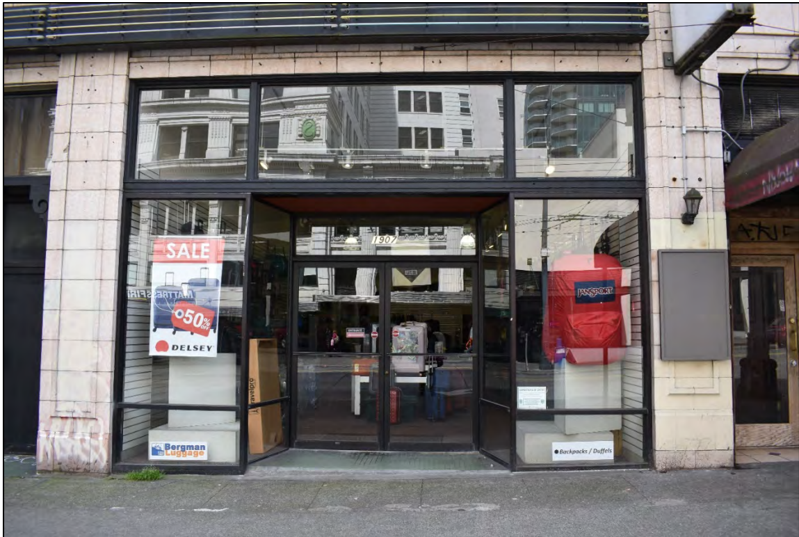
Fig. 17 – East elevation, detail of fifth bay, lower part, showing non-original storefront, typical
