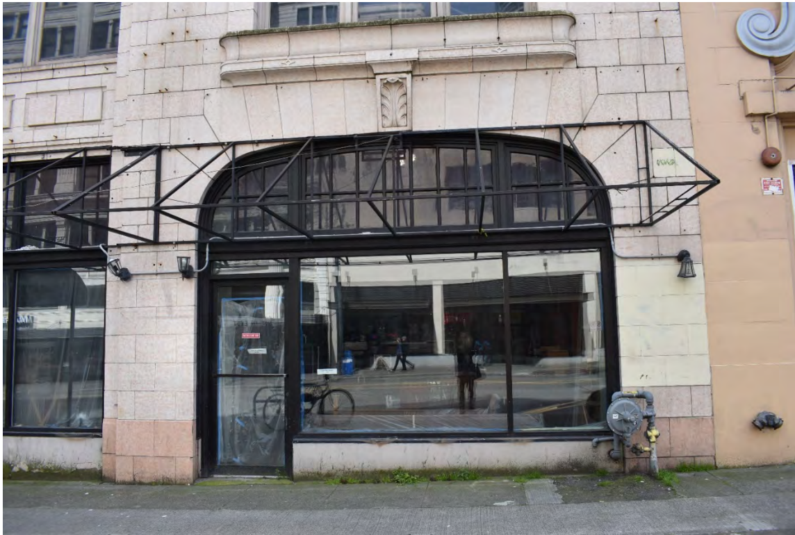
Fig. 15 – East elevation, detail of sixth bay, lower part
