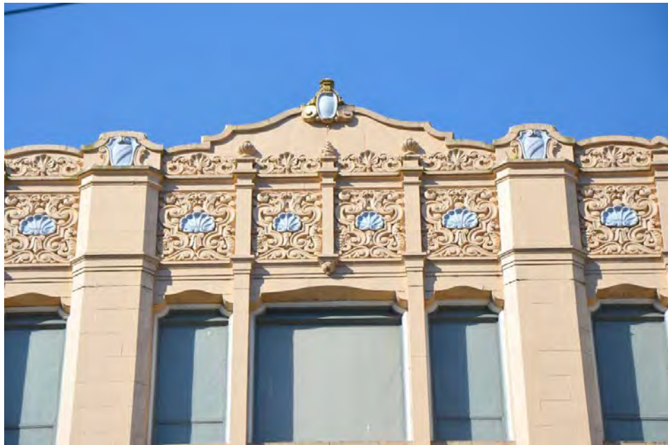
Fig. 86 – (Two images) White Garage (1928, Henry Bittman) at 1915 3 rd Avenue. The structure is a Seattle landmark, and adjacent to the subject building. (DON; SWCA Environmental Consultants)
