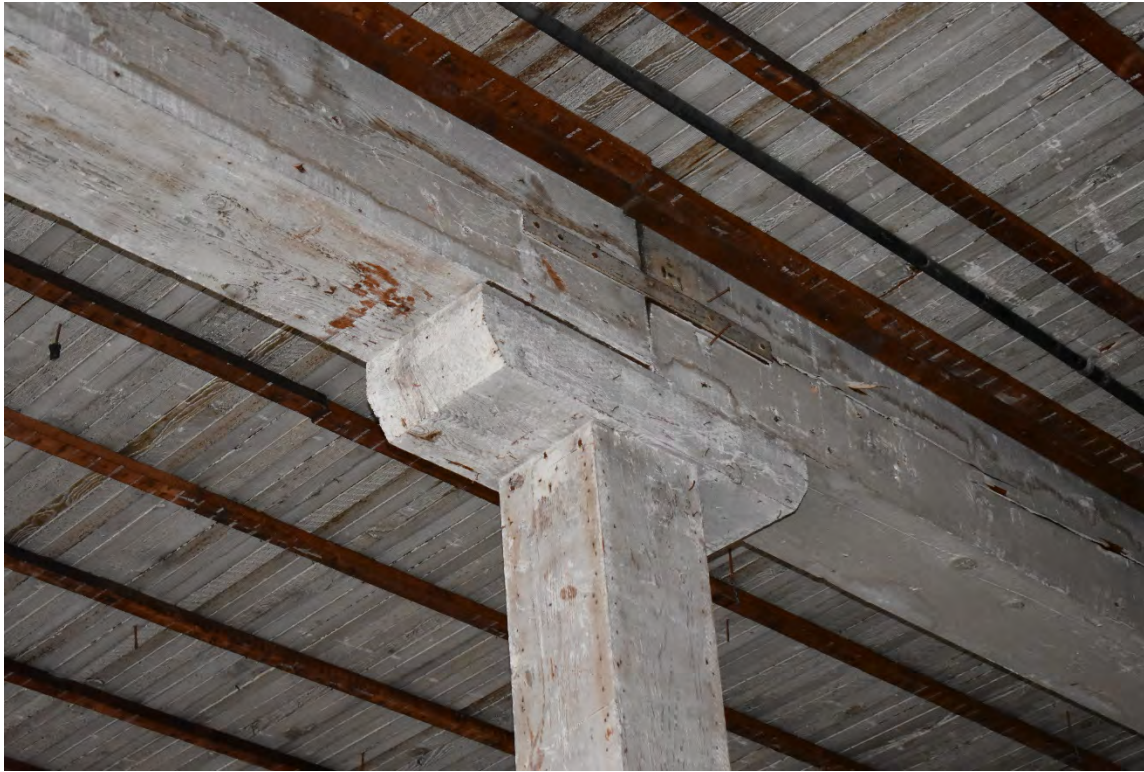
Fig. 33 – Interior, second floor, detail of post and beam
