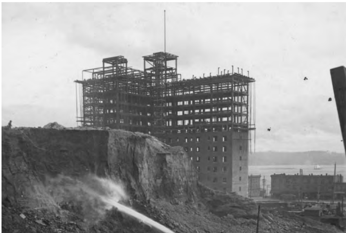
Fig. 43 – The New Washington Hotel (aka Josephinum Apts) under construction, c.1907-08, with regrading of Denny Hill still underway east of it. This would have been the surrounding conditions when Michael Donahoe bought the subject site.
