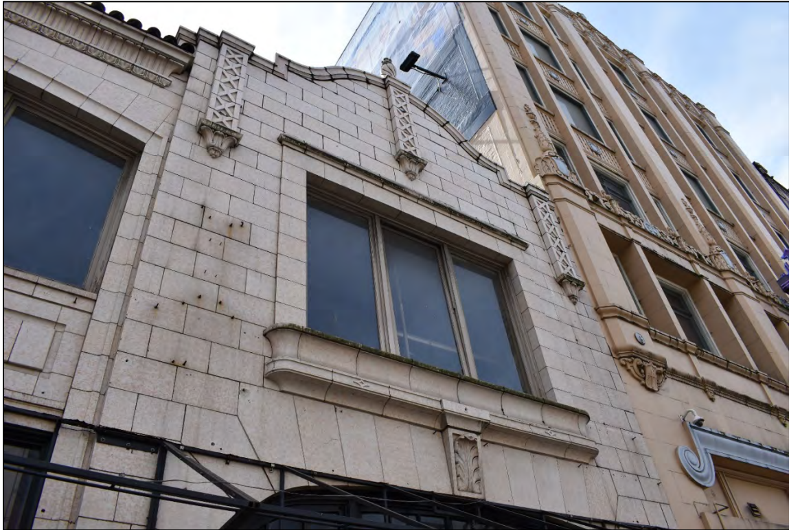
Fig. 14 – East elevation, detail of sixth bay, upper part. Window dates to between 1923 and 1937, likely installed during 1924 alterations.
