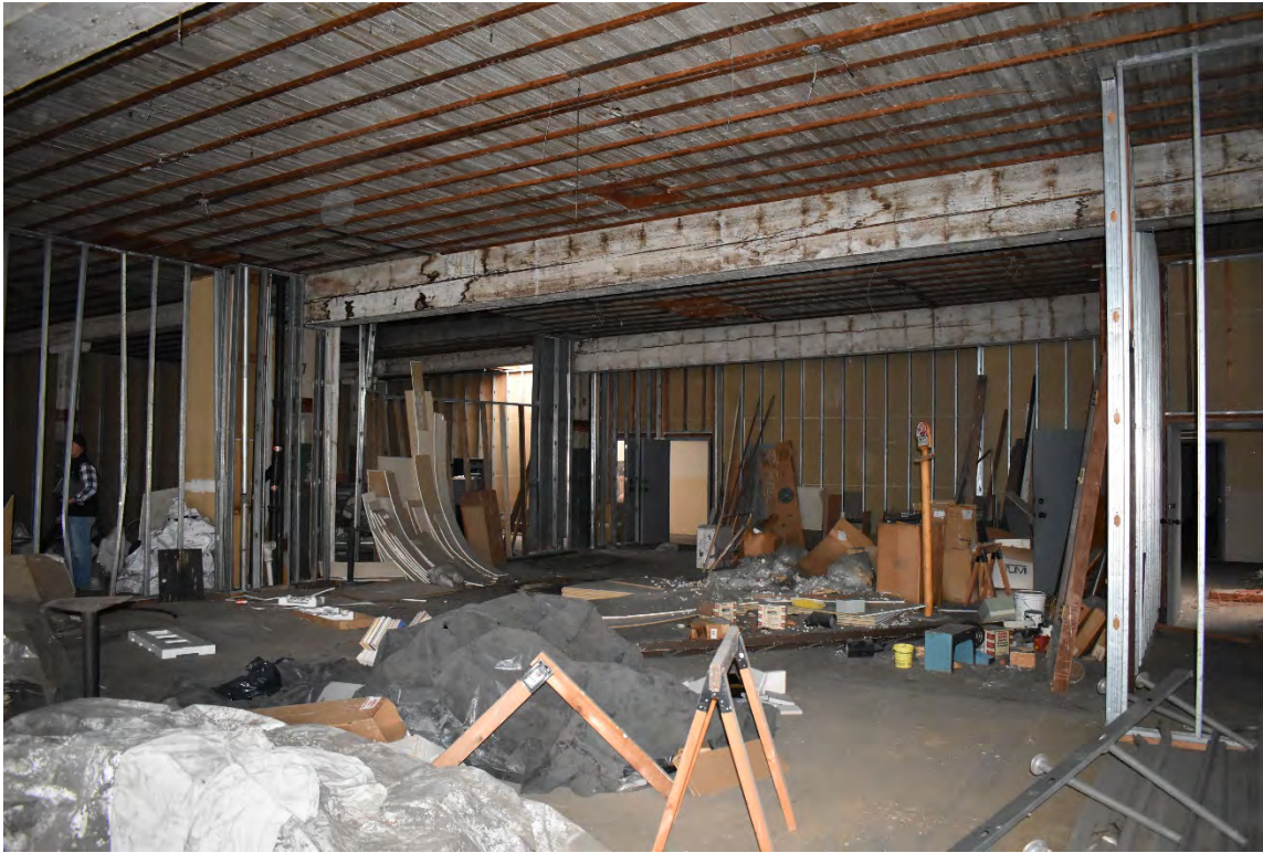
Fig. 31 – Interior, second floor, view towards middle of building
