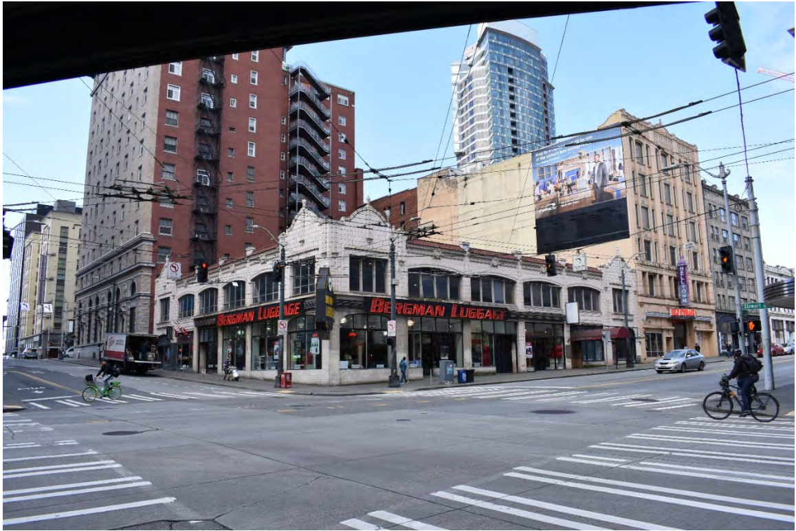
Fig. 7 – South and east elevation
