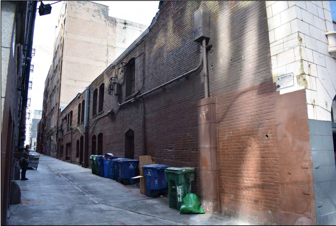
Fig. 19 – West elevation (alley), view north
