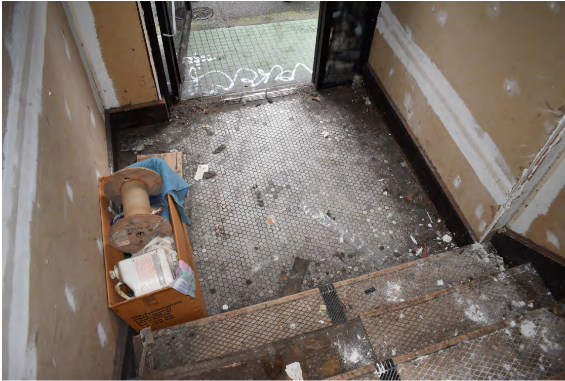
Fig. 29 – Interior, stairway to second floor, at third bay on 3 rd Avenue
