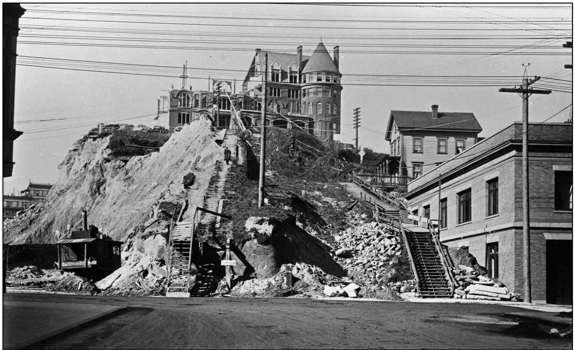
Fig. 41 – Circa 1905 view towards the Denny/Washington Hotel during demolition. 3 rd Avenue is yet to be cut through. The building corner at lower right corresponds now to the southwest corner of the Macy’s/Bon Marche department store. (Paul Dorpat)
