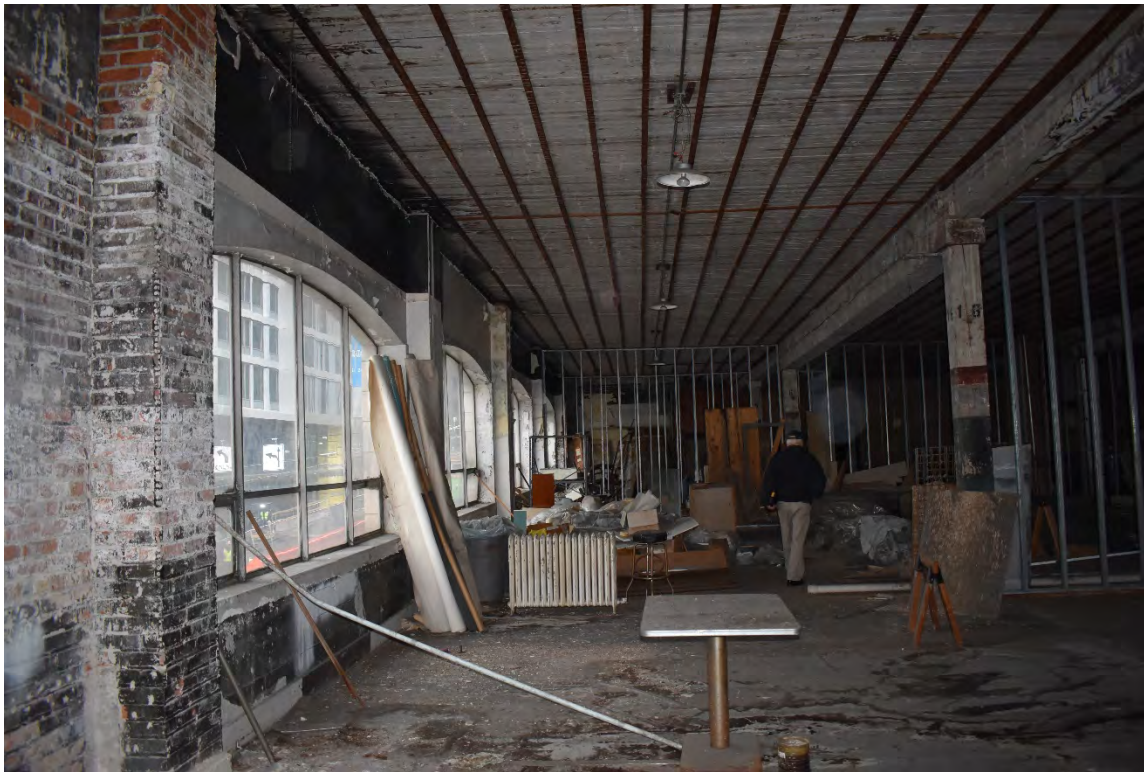
Fig. 30 – Interior, second floor, showing south elevation windows (Stewart Street)
