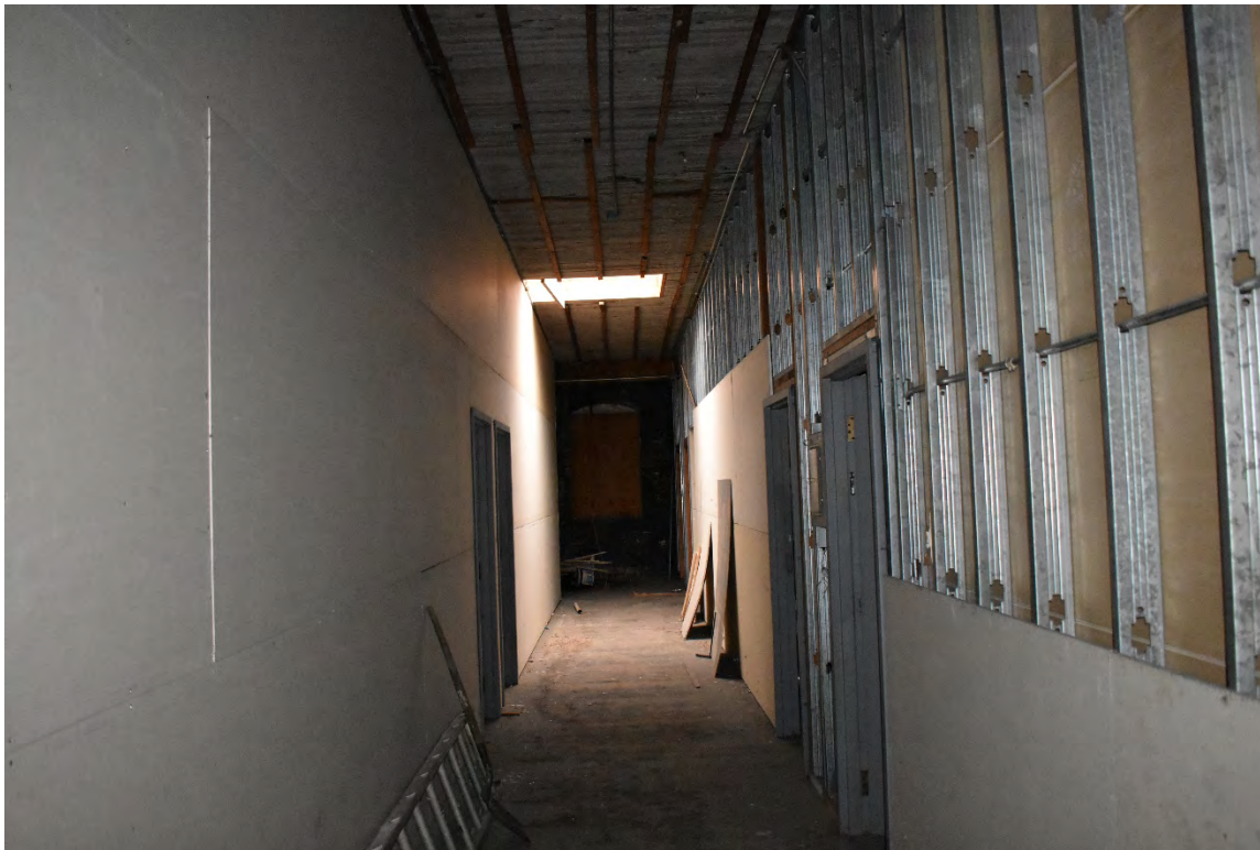
Fig. 34 – Interior, second floor, typical corridor with skylight
