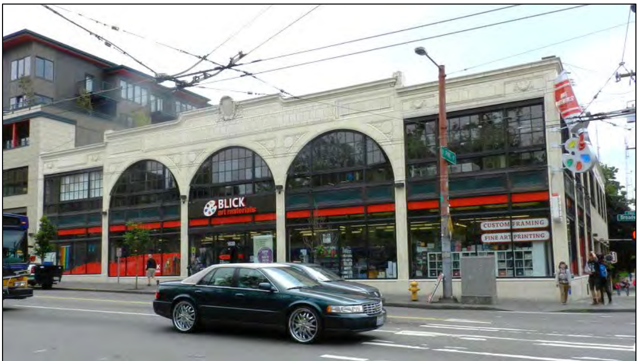
Fig. 57 – Comparable buildings: Boone & Co. Pontiac dealership (1925, altered) at Pine & Broadway. This building is clad in terra cotta. (DON)
