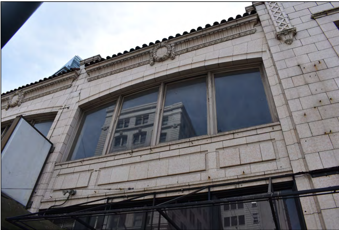
Fig. 16 – East elevation, detail of sixth bay, upper part. Window dates to between 1923 and 1937, likely installed during 1924 alterations.
