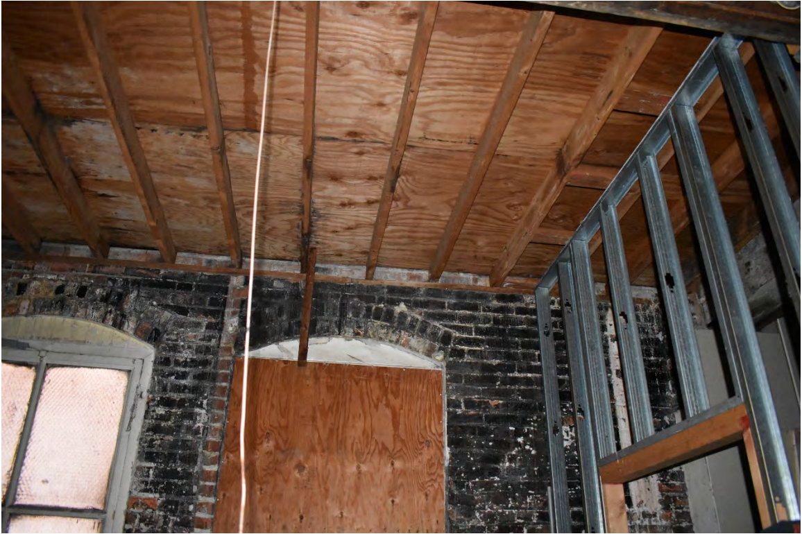
Fig. 35 – Interior, second floor, alley side showing repair at location where roof collapsed.
